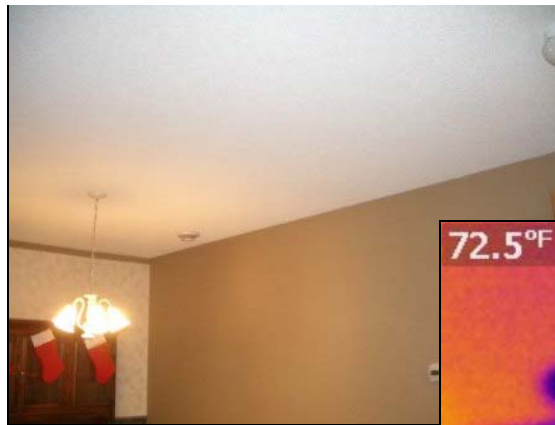
A water softener leak from the second story caused this wet area on the ceiling, which the homeowners disguised by re-texturing and re-painting. Mold growth is likely to occur in situations like this, so the sheetrock should have been replaced.
